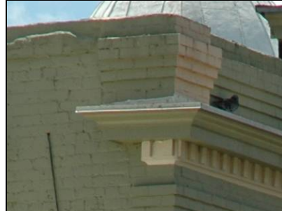
Note harder brick on the front façade and softer, secondary brick on the side façade or party wall, which requires gentle treatment if exposed.
