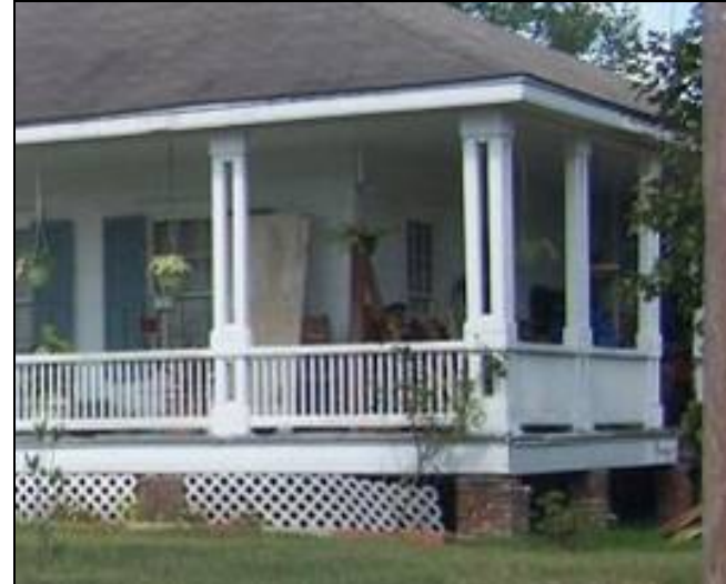
On this porch, the Lake Charles columns, brackets, and pedimented roof form are character-defining features of the Queen Anne Style and should be preserved.
