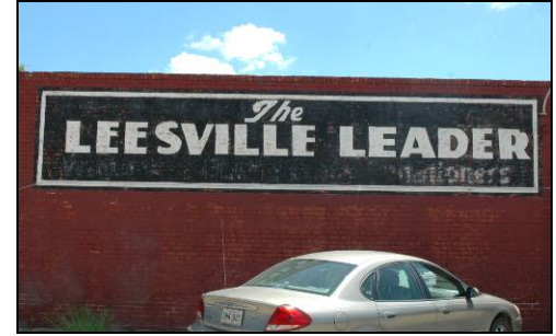
Original painted signs enhance the character of historic commercial buildings. Preservation or restoration of the paint should not trap moisture in the brick underneath.
