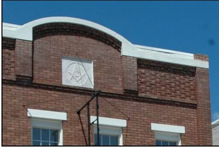
The character of an exterior wall is defined by its texture, color, and pattern. Note the textured brick and depth of the mortar joints.
