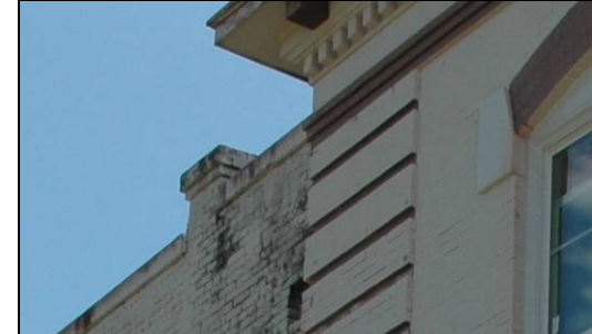
Note corbelled brick to simulate the appearance of quoins at the corner of the façade.
