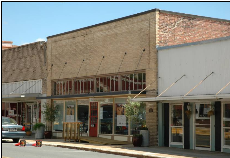
The metal canopies of these adjacent buildings are consistent in design and form and feature metal support rods. Note the canopies' subtle downward slope. Note how this central canopy runs horizontally between the transom above and the storefront below, so that it does not block any windows.
