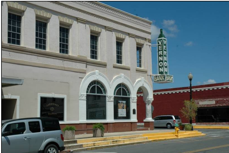
The stone detailing at the windows and roof cornice are character-defining features of this Renaissance Revival style building. Also note the historic signage.
