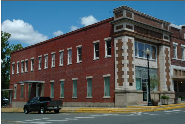
Example of a Renaissance Revival Style commercial building. Note the foundation details and decorative quoins at the front façade.
